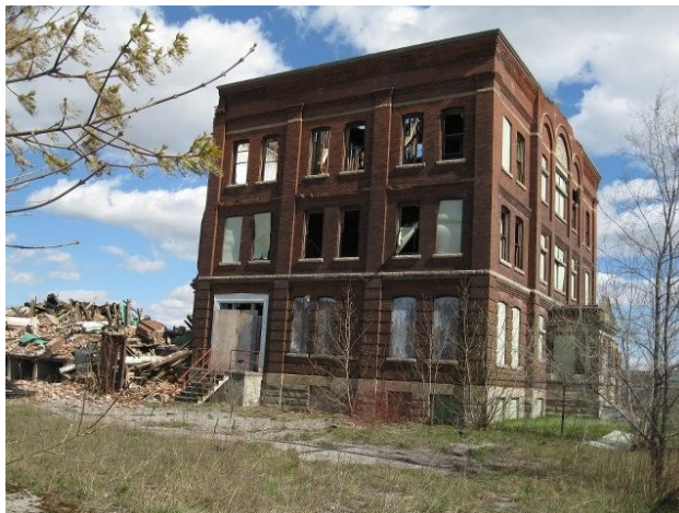
Cockshutt Office Building at 66 Mohawk in Brantford following fire. Photo by Mike Tutt
